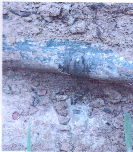
SPILL POINT DURING EXCAVATION:fig2
